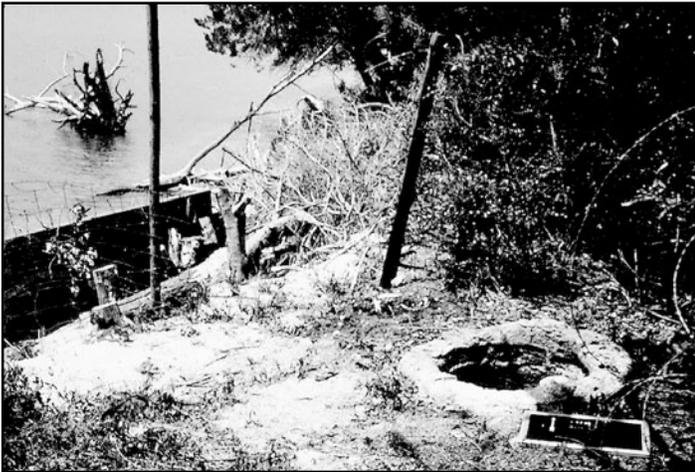
Riprap, or layers of stone placed along a shoreline to prevent erosion, and geo-webbing create a revetment for the Shell Bluff site.
