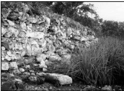
*Shoreline erosion of fort wall, Fort San Marcos de Apalache, before construction of a protective bulkhead.*
