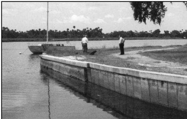
To the left is the seawall protecting the back face of Crystal River mound. A seawall is a structure separating land and water areas primarily to prevent erosion and other damage caused by wave action.
