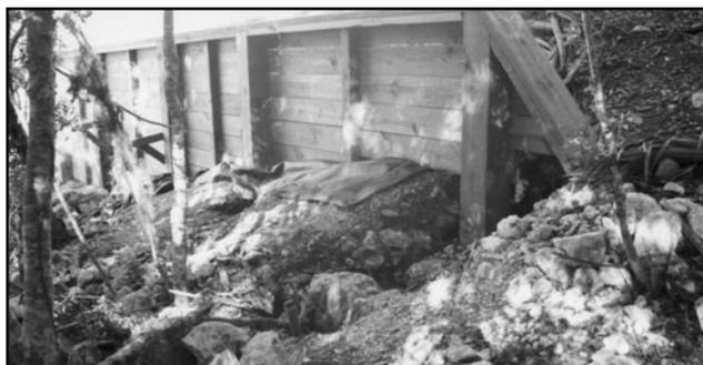
*A bulkhead is a structure that retains or prevents land from sliding into the water or protects it from wave damage. It functions much like a seawall (see Crystal River case study for seawall illustrations).*
