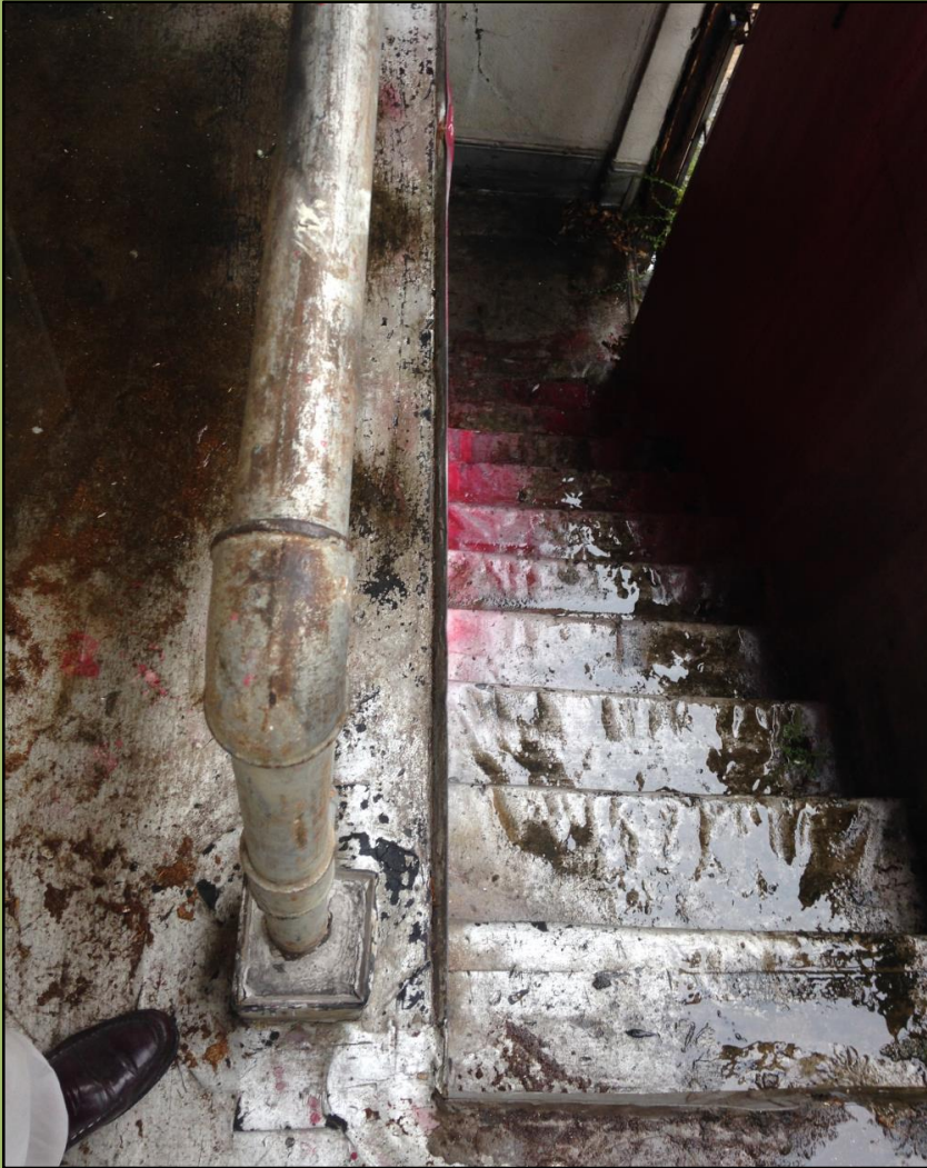
#1 Stairwell and railing condition 11/2015 Pre-rehab
