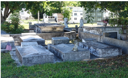
Above ground features and vaults like these in the Key West Cemetery can become dislodged or flooded from storms or increased inundation.
