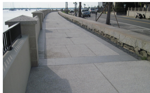
A new seawall built in St. Augustine included preservation methods for the historic seawall shown along the right side.
