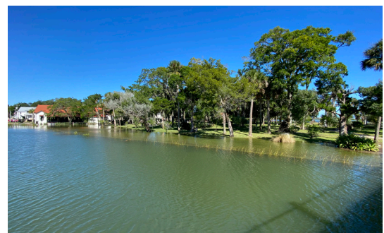
Pond feature overtopped and encroaching into St. Augustine’s Sacred Acre near La Leche site.
