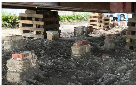
Studying foundations during a flood mitigation project can reveal new information such as foundation systems from previous buildings.
