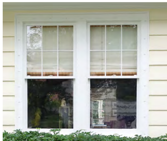
Traditional window pattern with six lites (lights) on the upper sash and one below.
