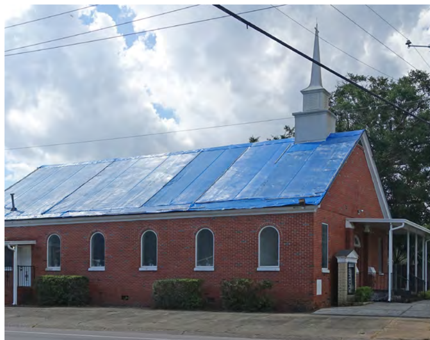
Blue roof tarps are a common following a hurricane or other strong wind event and should only be temporary solutions.
