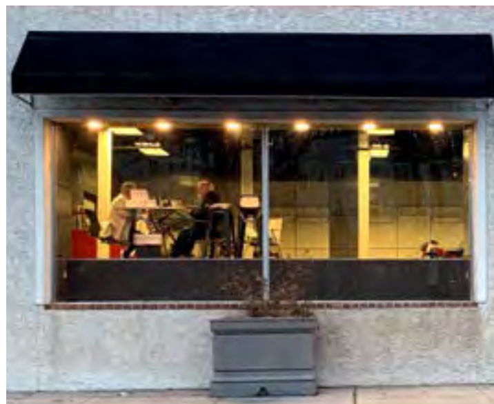
The interior floor has been elevated above the DFE at this former warehouse.
