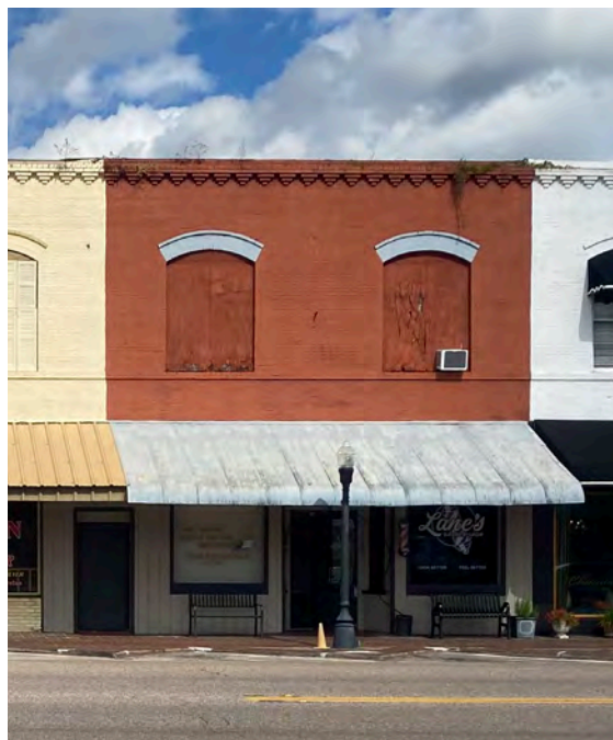
Plywood panels can be painted to blend with the adjacent wall surface if installed for a long period of time after a storm.
