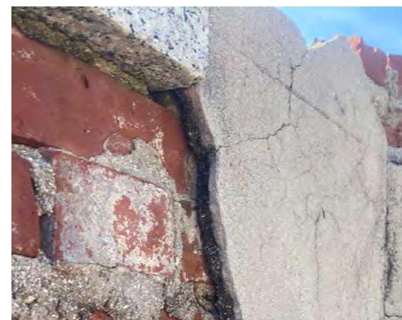
Masonry buildings may have multiple components that can separate and allow water intrusion making them poor candidates for dry floodproofing.
