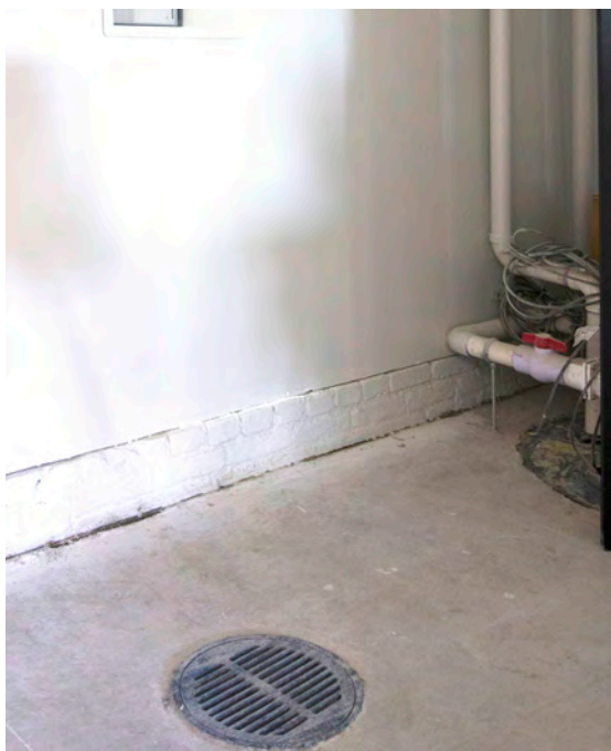
Flood water seepage collected in the floor drain is removed by the sump pump at the right side of the photograph.
