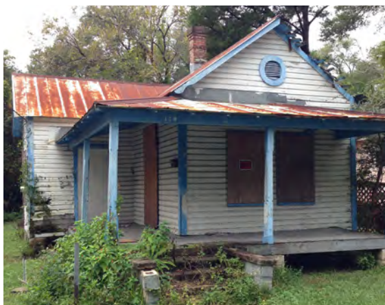
This early wood frame vernacular building has wood siding, wrap-around porch, and a metal roof.
