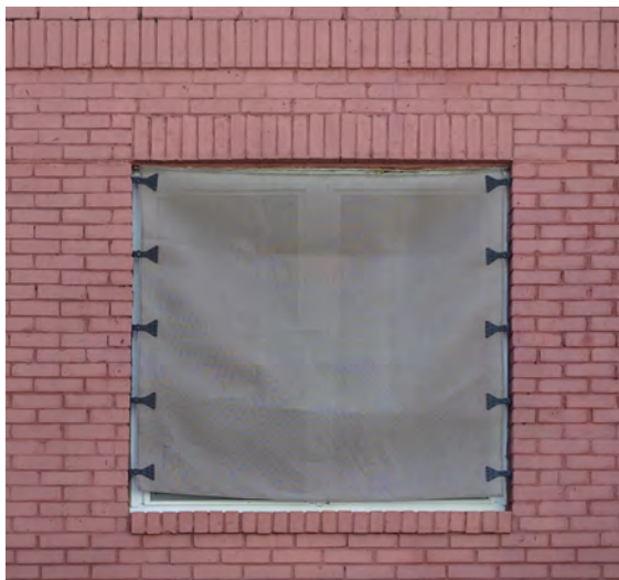
Fabric panels are an option for temporary protection that can be easily stored.
