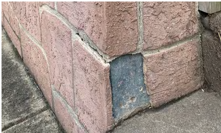
There are various types of stone and veneers used in Florida's historic buildings that need to be inspected to ensure they are not separating from the wall.
