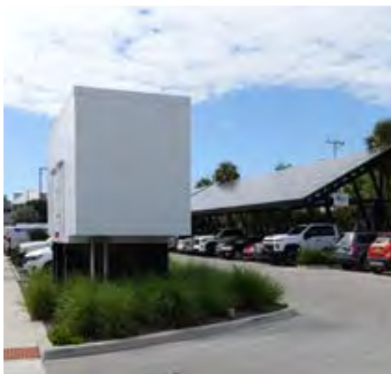
Solar panels located on the parking shade structure in the Key West City Hall parking lot and a large generator is raised above the parking median. The secondary power sources provide electricity to City Hall when needed.
