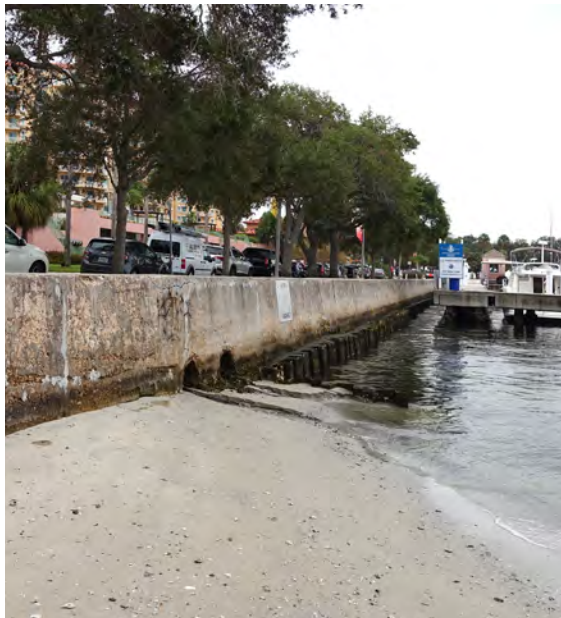
Bulkheads act as retaining walls at the water's edge. They may not provide storm surge protection and are often inadequate to address sea level rise.
