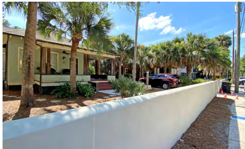
Multiple property owners cooperated to build a front property wall with driveway door dams that can be installed in advance of a severe storm.
