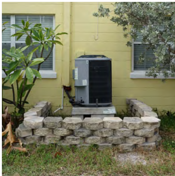
Elevating mechanical systems is recommended and can reduce flood insurance costs.
