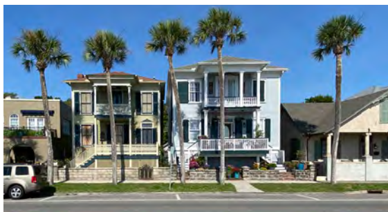
Two adjacent buildings were elevated to different heights.
