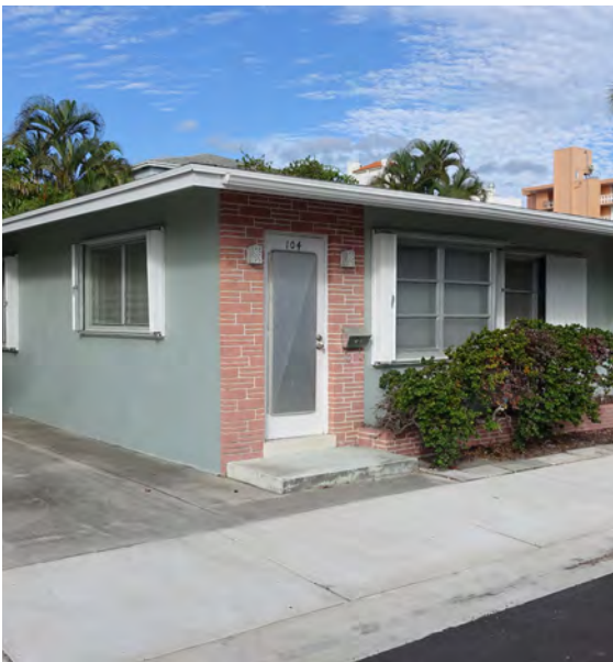
Homes with flatter roofs may have wider eaves or overhangs as part of the roof structure.
