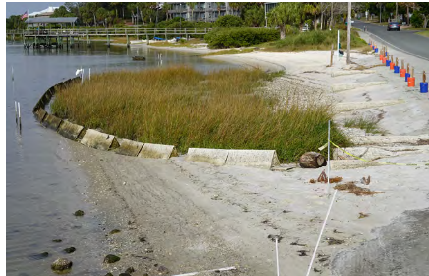
Living shorelines, which include marsh grasses and mangrove stands, can reduce the impact of storm surge. In this example, concrete barriers protect the marsh grass as the roots become more established and take hold.
