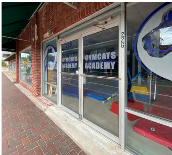
Historic commercial buildings often have aluminum storefronts. The large windows and glazed doors are highly vulnerable to air-borne debris. Glass protection and enhanced hardware can improve wind resilience.
