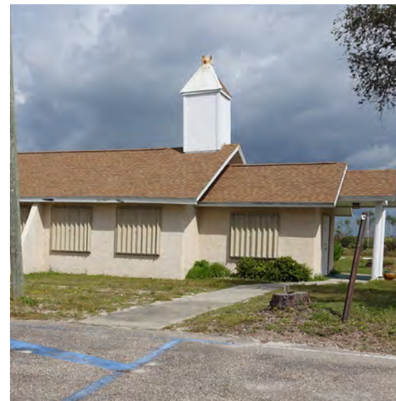
The best option for some properties are hurricane shutters. They should remain open when not needed for protection.
