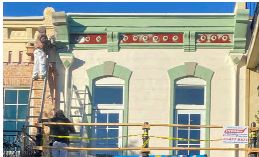
Paint is decorative and also a surface finish that needs to be maintained to protect the historic materials underneath from environmental damage.
