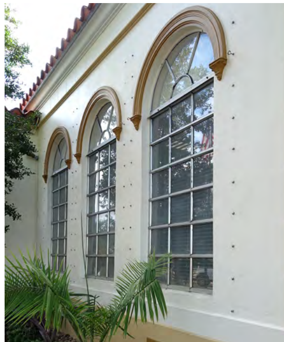
Fasteners may need to be permanently installed to allow proper anchoring of window protection.
