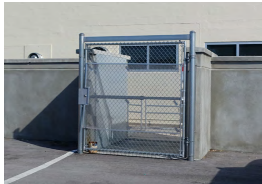
A high school in Everglades City uses a concrete perimeter wall and a flood gate that deploys with the rising flood waters.
