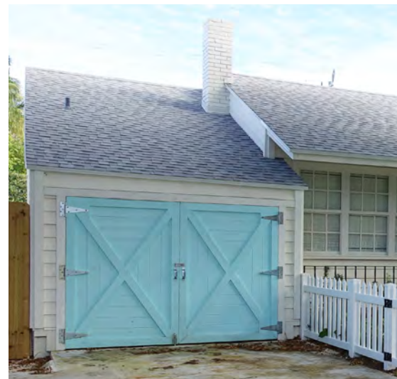
Garage doors are more historically more prevalent at post-WWII buildings. Historic wood doors can be reinforced from the interior to improve wind resilience.
