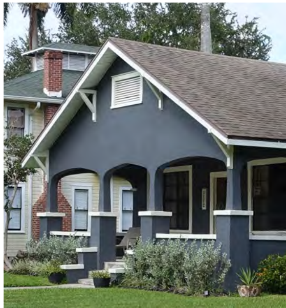
Gable vents in older homes allow attic ventilation and are not just decorative features.
