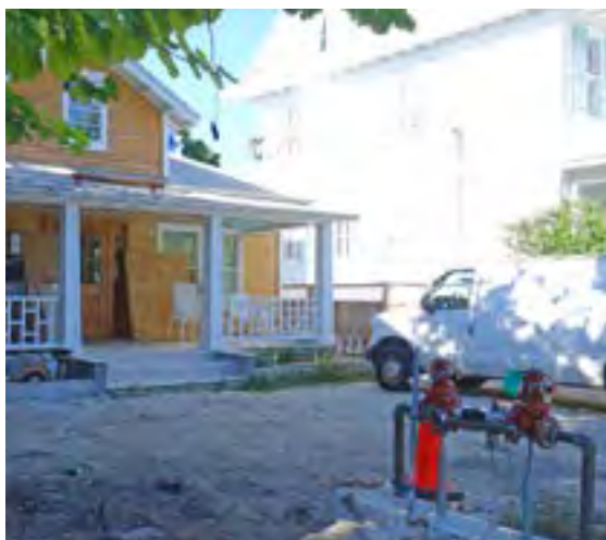
Local regulations may require locating back flow preventers close to the city utility lines.
