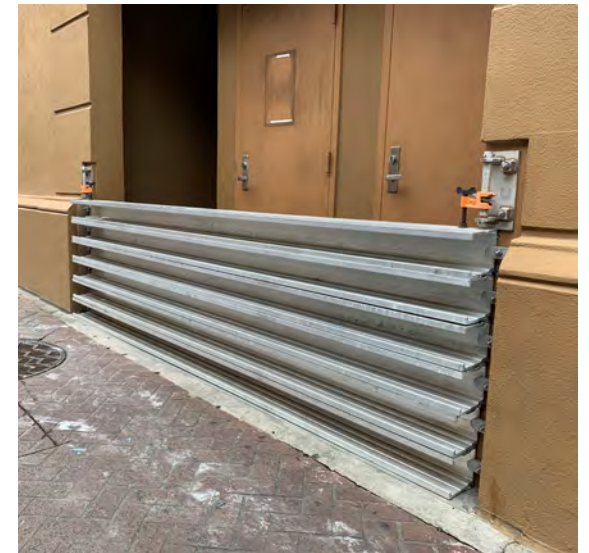
Large-scale Dry Floodproofing measures must be engineered to withstand the force of flood water.
