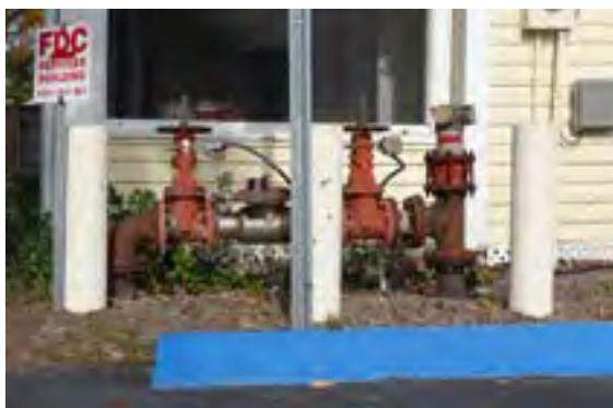
Commercial scale back flow preventer systems are larger than residential systems.
