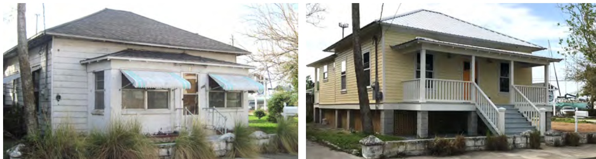
A residence before and after elevation. As part of the elevation, the original open front porch was restored, steps were maintained on center with the entrance door, and unobtrusive foundation screening was added at the rear of support piers.
