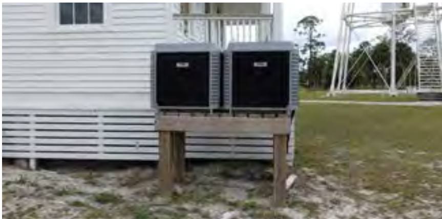
Elevated utilities can be screened with landscaping or fencing. Provide access for ventilation and maintenance.
