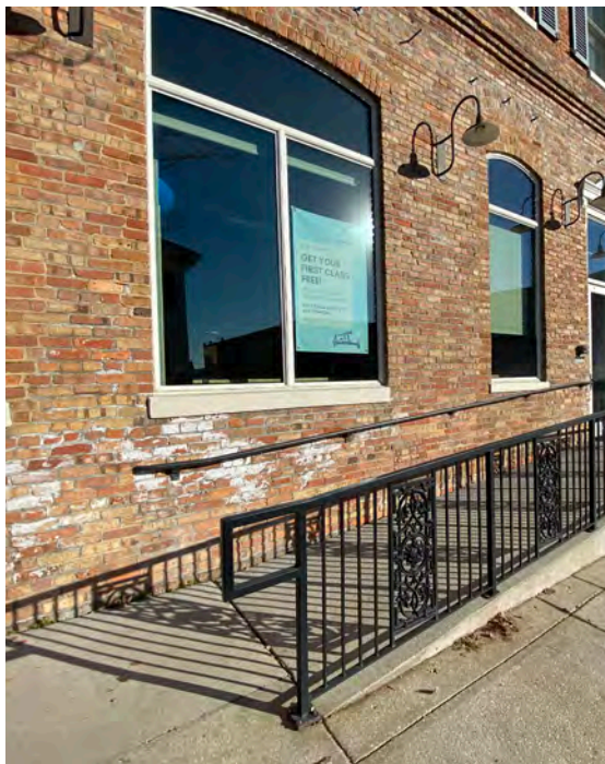
This corner commercial building in Pensacola's downtown had a sidewalk wide enough to install a ramp on the side elevation. The ADA establishes the requirements for the ramp slope, width, handrail height, and handrail configuration.
