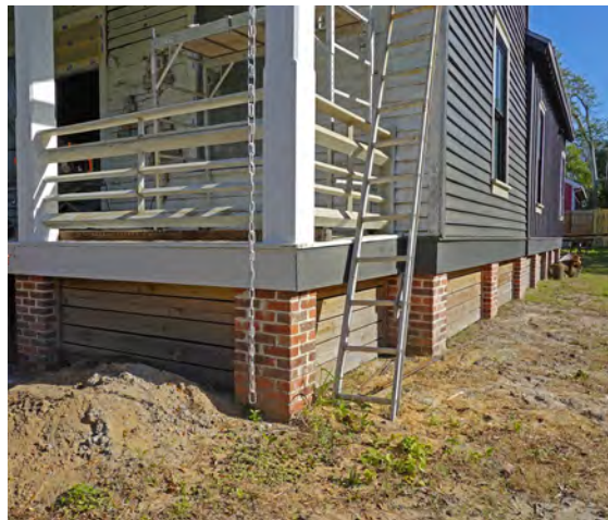
Horizontal boards are recessed from the front plane of the foundation piers.
