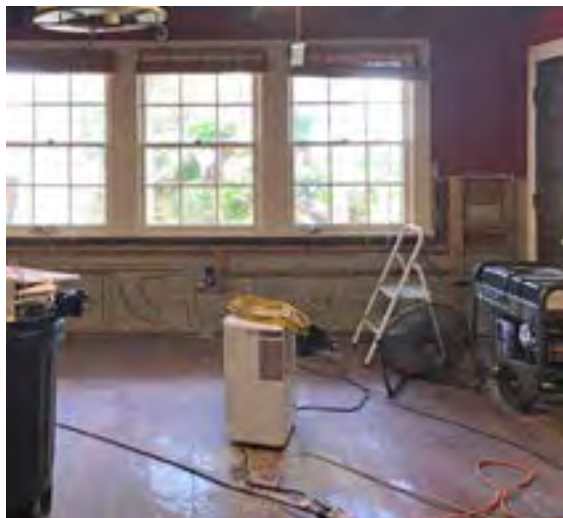
Cleaning and drying out interior spaces should be conducted methodically to salvage historic finishes.
