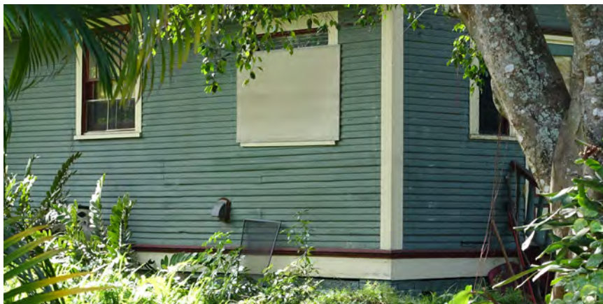
Failing paint and moisture can contribute to the deterioration of wood siding and should be repaired as soon as possible to avoid a larger repair project.
