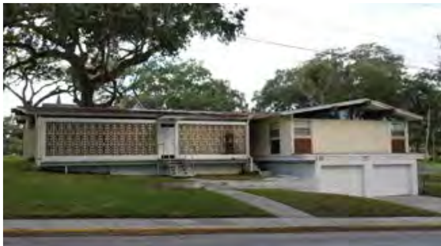
Areas at lower levels of wet floodproofed buildings may only be used for parking, storage, and building entrances.
