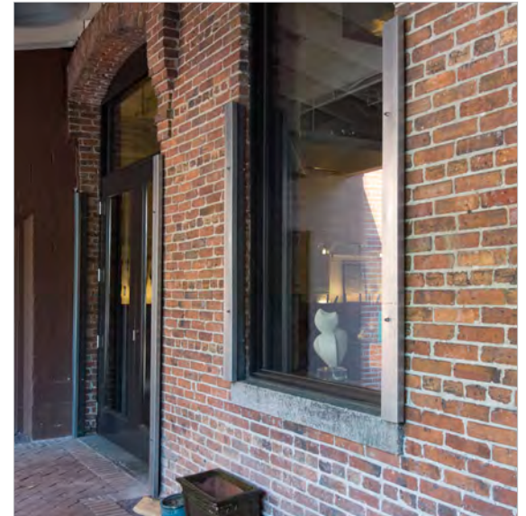
The metal frames flanking the window and door openings are used to hold flood barriers in place.
