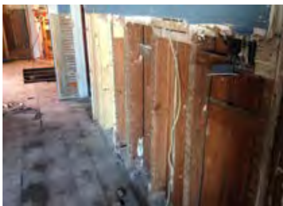
Removable baseboards may allow ventilation and reduce damage to historic finishes.
