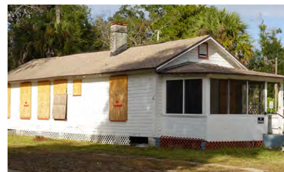
Plywood is often the most flexible and affordable choice for window protection.
