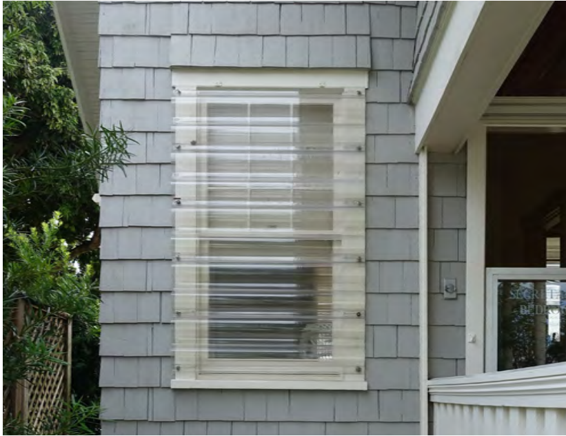
Lucite hurricane panels are temporary solutions installed prior to a storm event leaving only fastener anchors visible when coverings are not in use.
