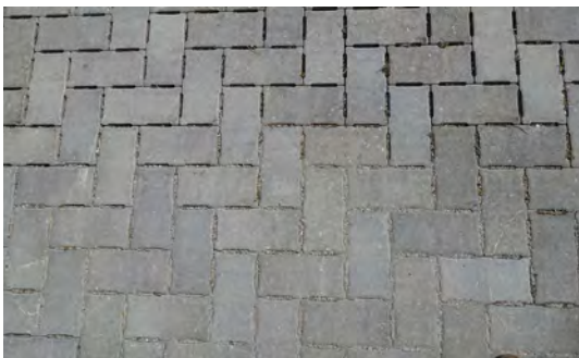
A variety of permeable pavers have been developed that can look like traditional brick.
