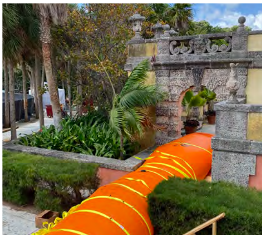
Vizcaya, located in Miami, uses deployable barriers to protect its historic architectural and landscape features from flooding. (Courtesy of Adrienne Burke)
