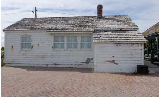
Building maintenance can reduce potential damage from heavy rain and winds.
