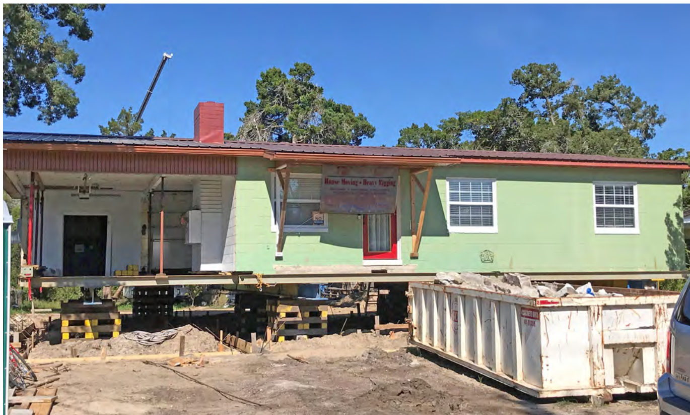
Building elevation can have a significant impact on the historic appearance of a building.
