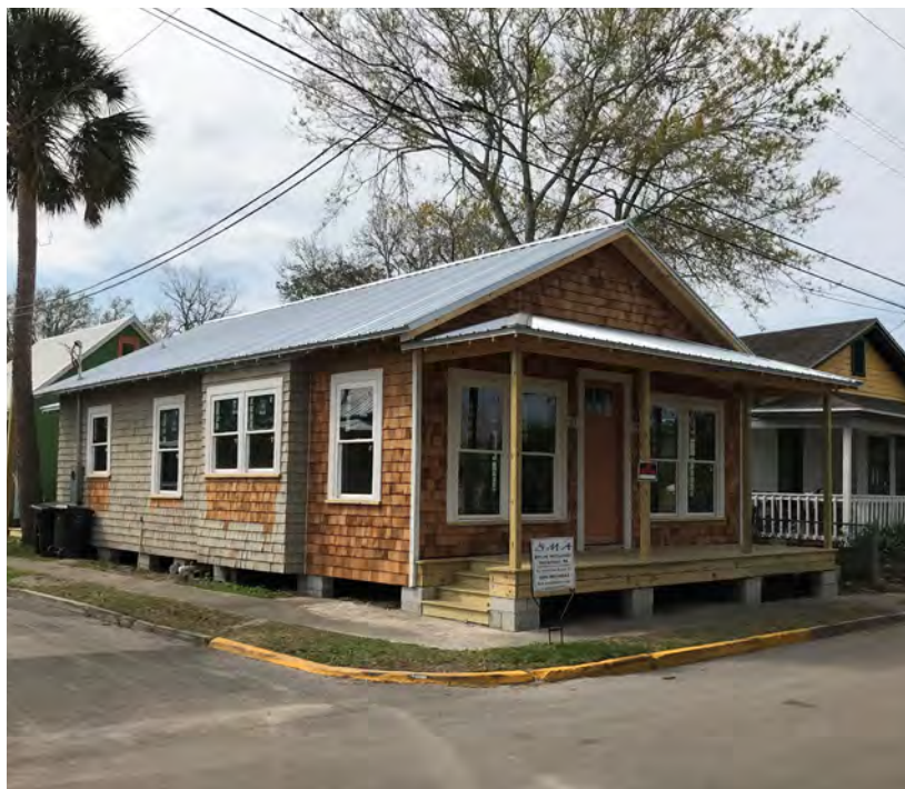
A variance was issued when this building underwent rehabilitation allowing the finished floor elevation to remain unaltered.
