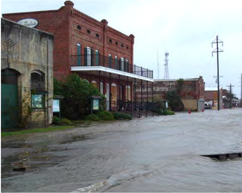
Hurricane Dennis, 2005, flooded Apalachicola streets and vulnerable historic commercial areas.
