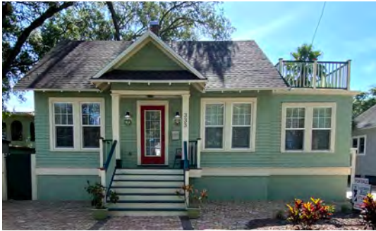
After Elevation: A compatible design should be carefully chosen for the newly constructed foundation wall.
