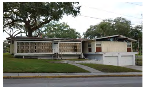
Basements are not common in Florida but may be found in areas with elevation changes on site.
