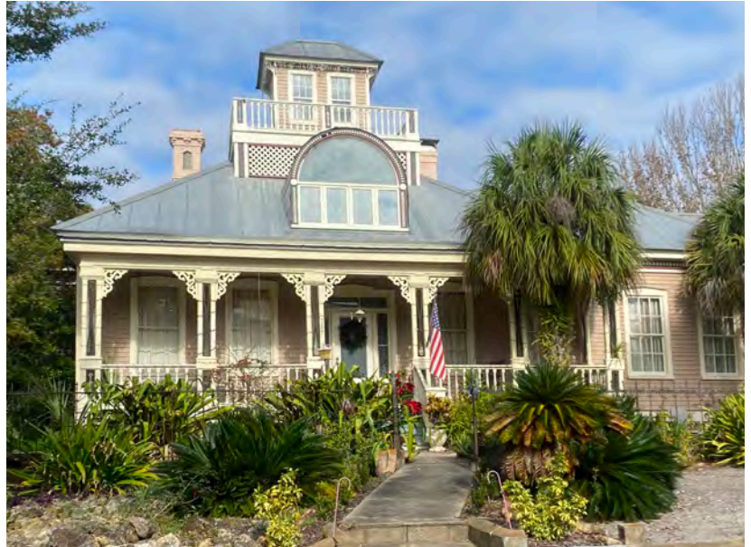
Historic buildings may have more complicated roof systems with attached roof features that will require a careful mitigation plan.
