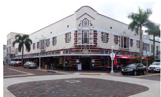
Paved areas can be converted to permeable pavers to reduce stormwater runoff.
