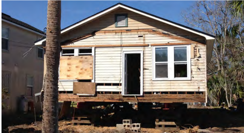
Property damage from a storm event can reveal other building weaknesses.
