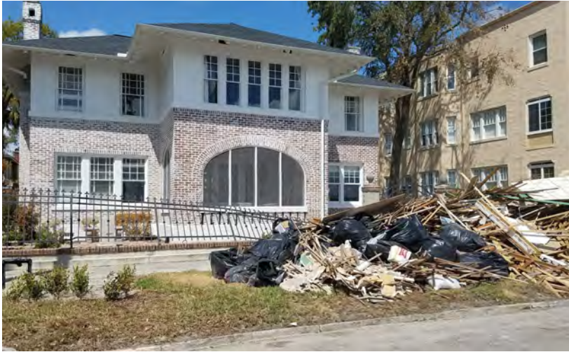
Flood damage can be extensive to interior finishes and furnishings. (City of Jacksonville)
