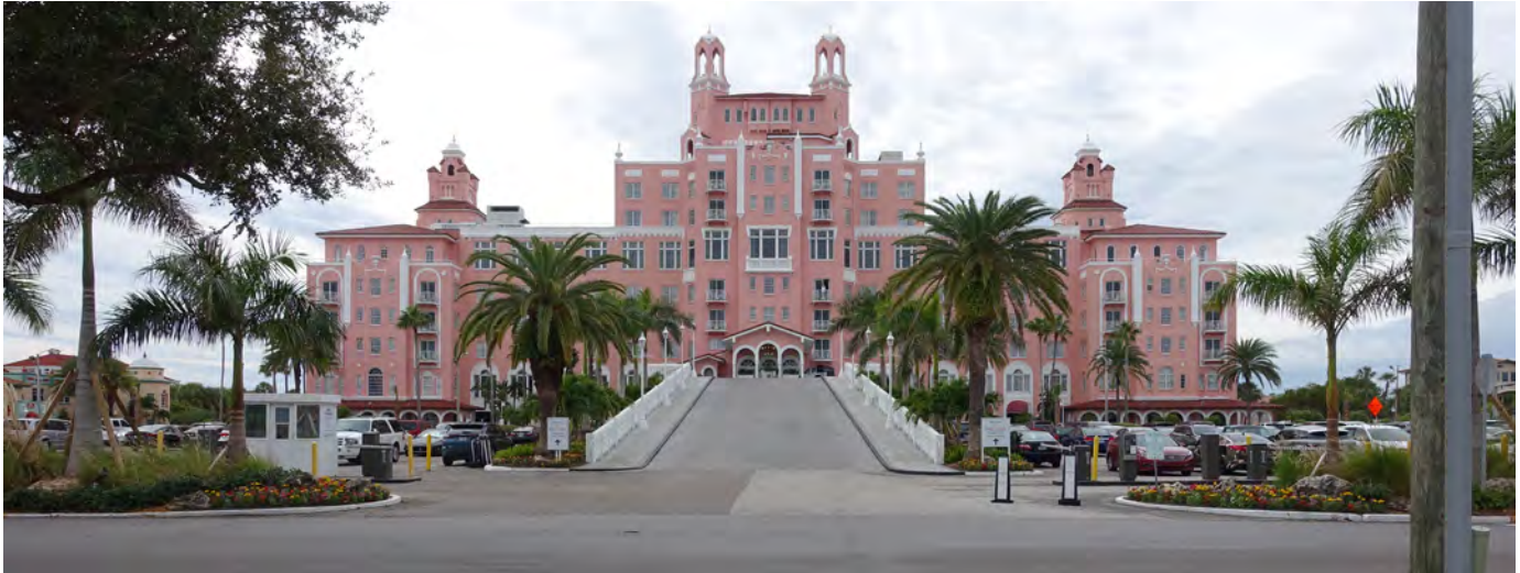
The historic Don CeSar Hotel in St. Pete Beach is situated in a flood zone.
