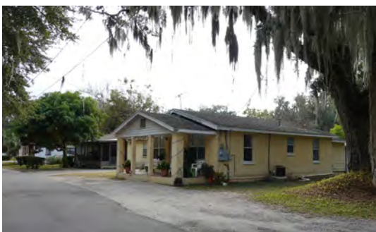
Areas without street infrastructure can be more vulnerable to flooding.
