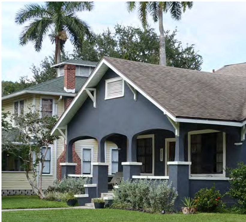
Gable vents in older homes allow air ventilation and are not just decorative features.
