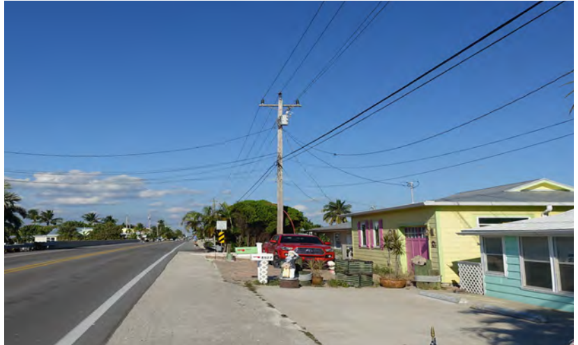
Emergency evacuation routes that are improved by raising the roads can cause additional stormwater impact to building below the new roadway height.
