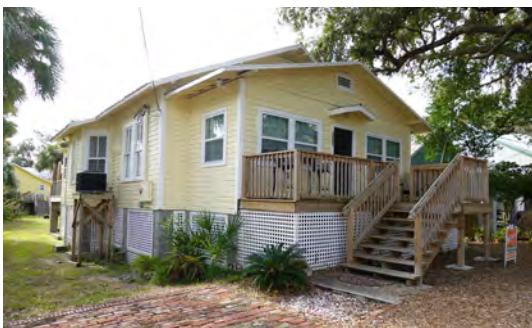
Most communities use the standard Base Flood Elevation requirement or additional freeboard.
