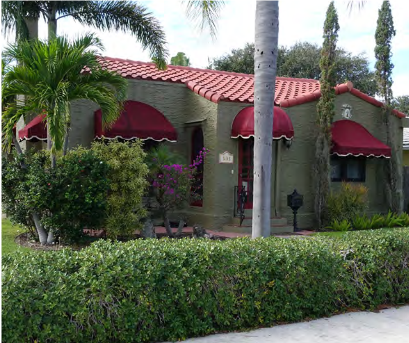
Historic Mediterranean Revival buildings usually have clay tile roofs that can cause challenges when seeking new insurance coverage.
