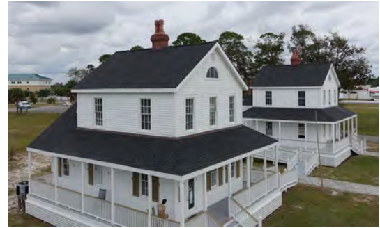
The Cape San Blas Lighthouse and Keeper's Quarters were relocated to Port St. Joe to reduce the threat of erosion, flood, and wind damage.
