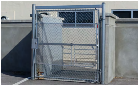
Permanent perimeter walls and floodgates are engineered to keep floodwater away and may be effective for groupings of buildings or significant large buildings.
