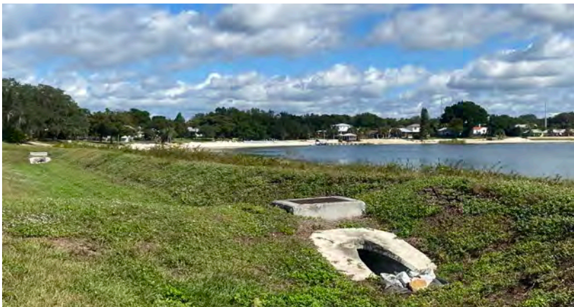
Stormwater retention areas can collect water and allow it to drain slowly while being filtered to reduce pollutants into natural waterbodies.
