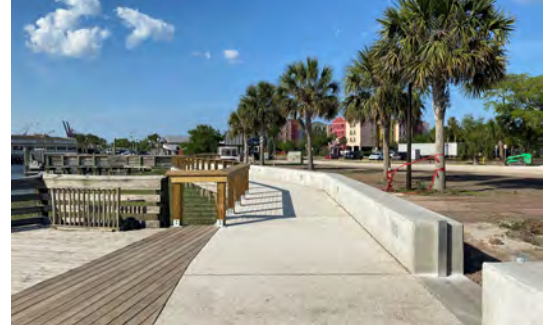
Seawalls are a common and traditional approach for community-wide mitigation strategies.
