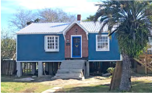
Reducing flood risk can mean changing access to individual buildings and its orientation on a lot.
