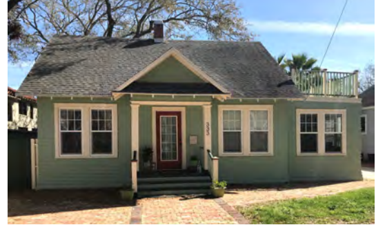
Prior to Elevation: Buildings on continuous foundation walls or piers are usually good candidates for elevation.
