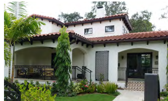
Clay tile roofs are important features that can be lost due to insurance company requirements.
