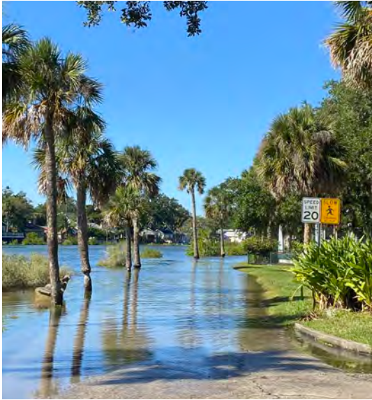
Future mitigation projects planned with input from the preservation staff will address flooding to historic buildings around Lake Maria Sanchez in St. Augustine as part of a larger DEP grant program.
