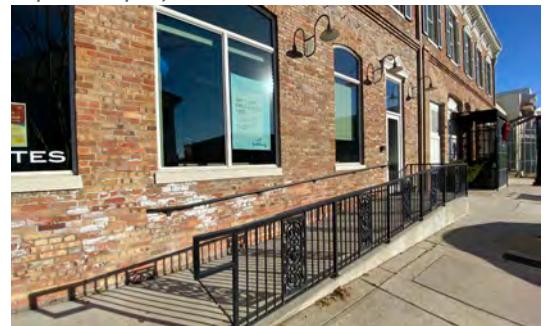
ADA requirements can be sensitively included during flood mitigation projects.
